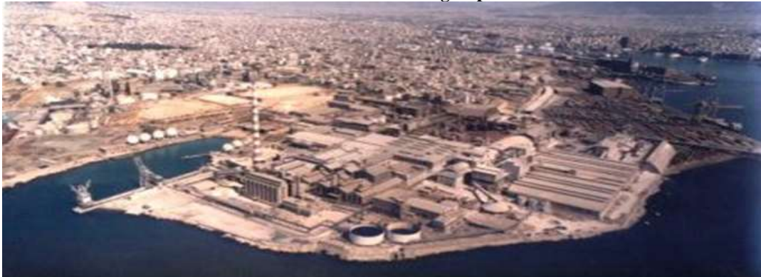
Figures 2a and 2b. The area that was occupied by the old Fertilizers Factory: before and after the demolition of its largest part.
